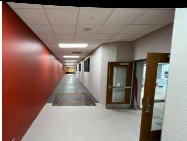
Corridor & Cafeteria Entrance
